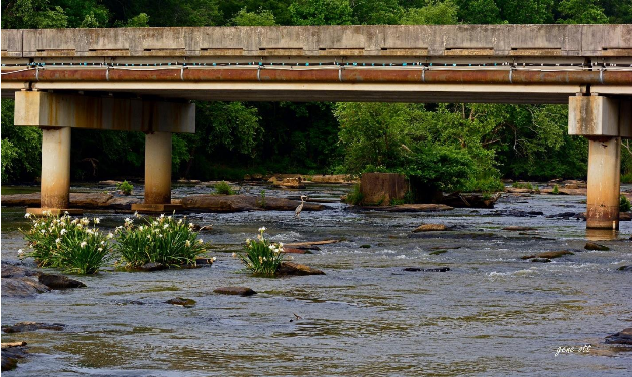
Figure 10. Bridge across shoals to Town of Ware Shoals, SC.
