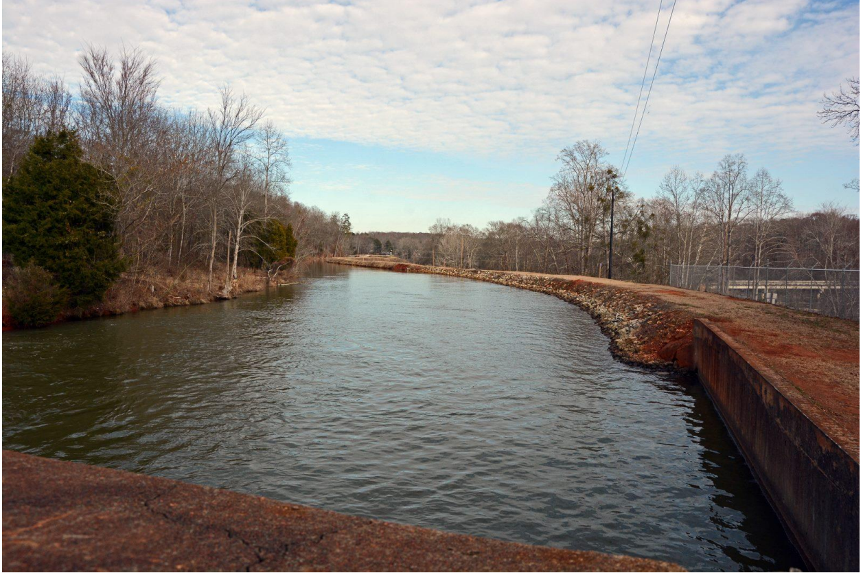
Figure 3. The aqueduct that transports water diverted to the powerhouse over a half-mile away.
