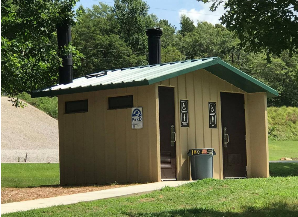
Figure 9. Toilet facilities at Irvin Pitts Memorial Park.
