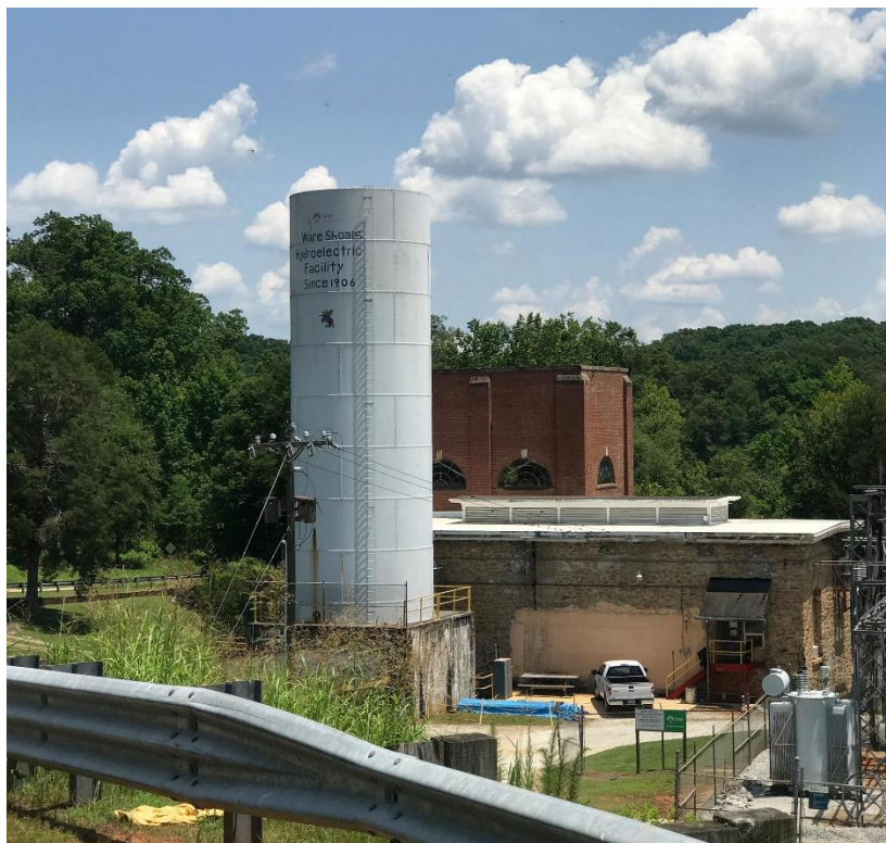
Figure 4. Powerhouse on Saluda River at Ware Shoals, SC.
