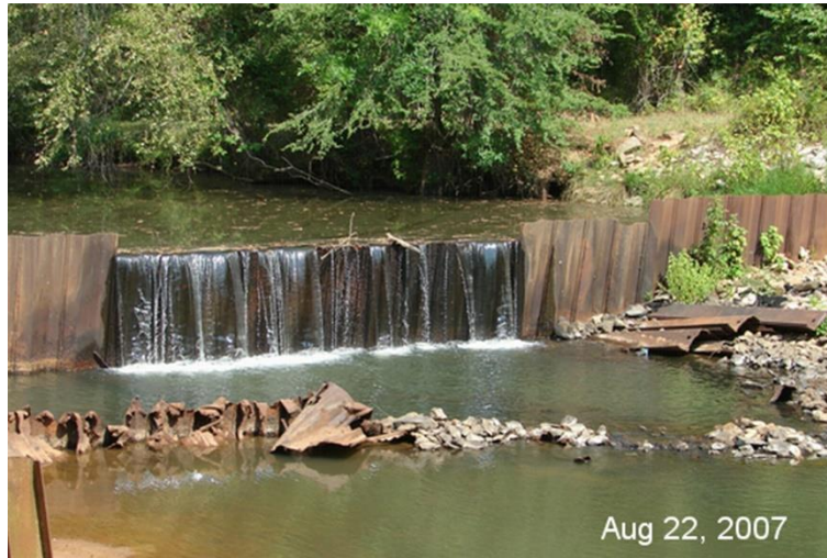
Figure 2. Cofferdam on Rabon Creek.
