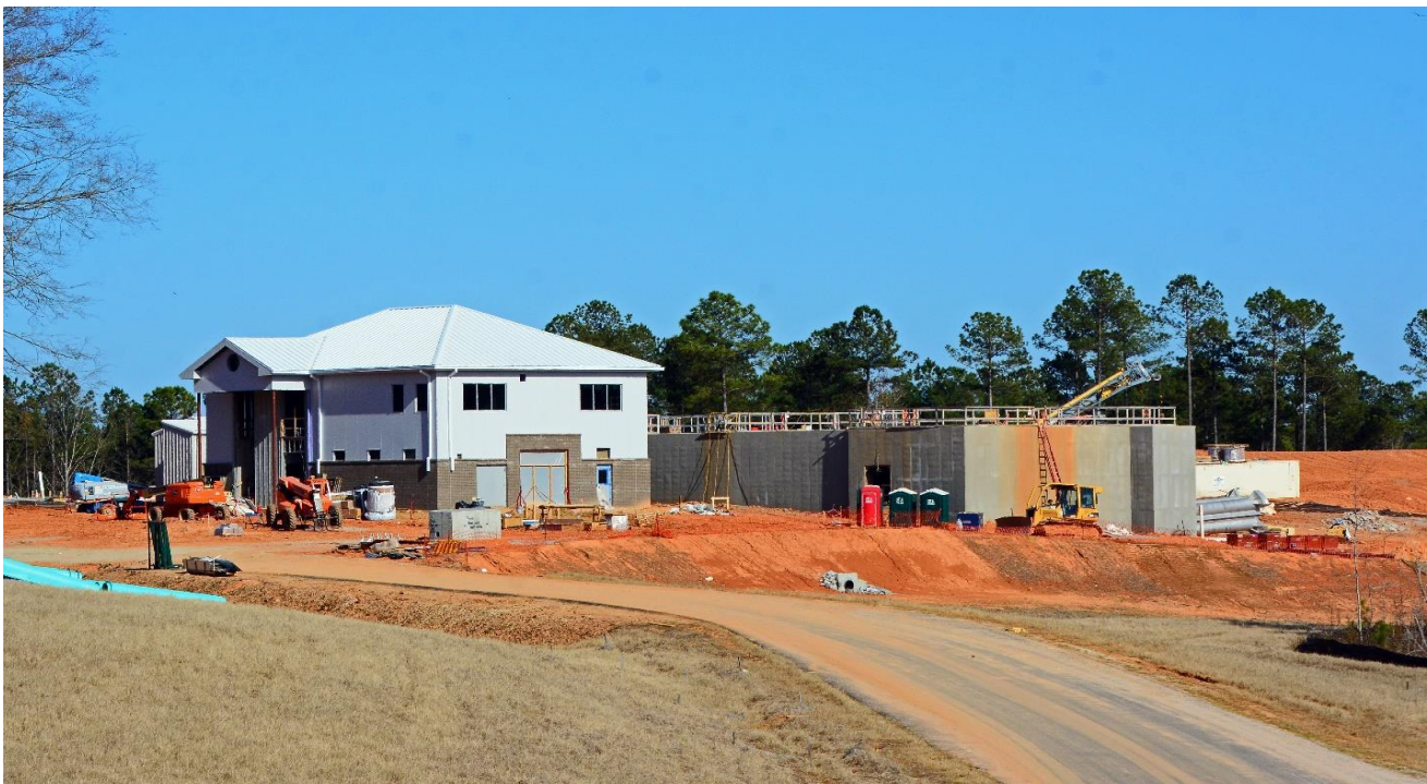
Figure 3. LCWSA Water Treatment Plant under construction.
